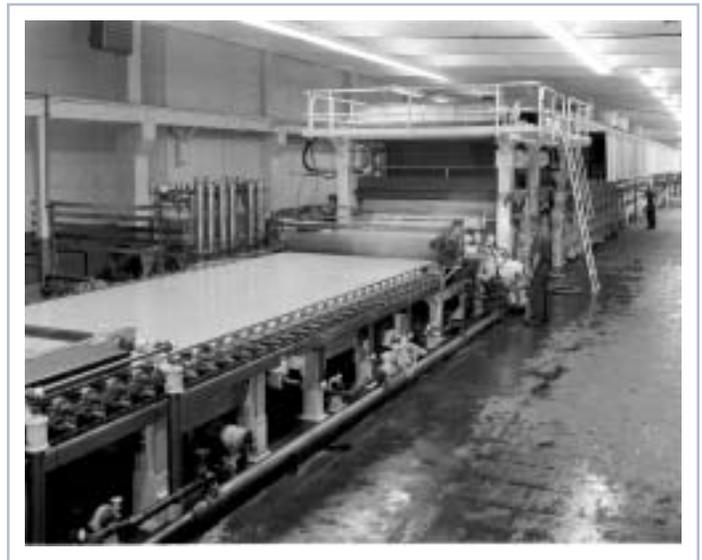
*A Fourdrinier paper machine at Strathmore Paper's Woronoco mill in Massachusetts circa 1950: To the left, pulp is dispersed into the wire where water is shaken out of the pulp to form the sheet or web of paper. The web continues through the press section and into the dryer. Then it is wound into large rolls which are later sheeted.*
